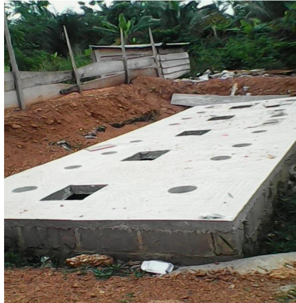
De septic tank van 9x3x3 m is gereed.
